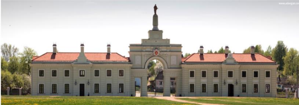
Restoration of the palace and park ensemble in Ruzany
