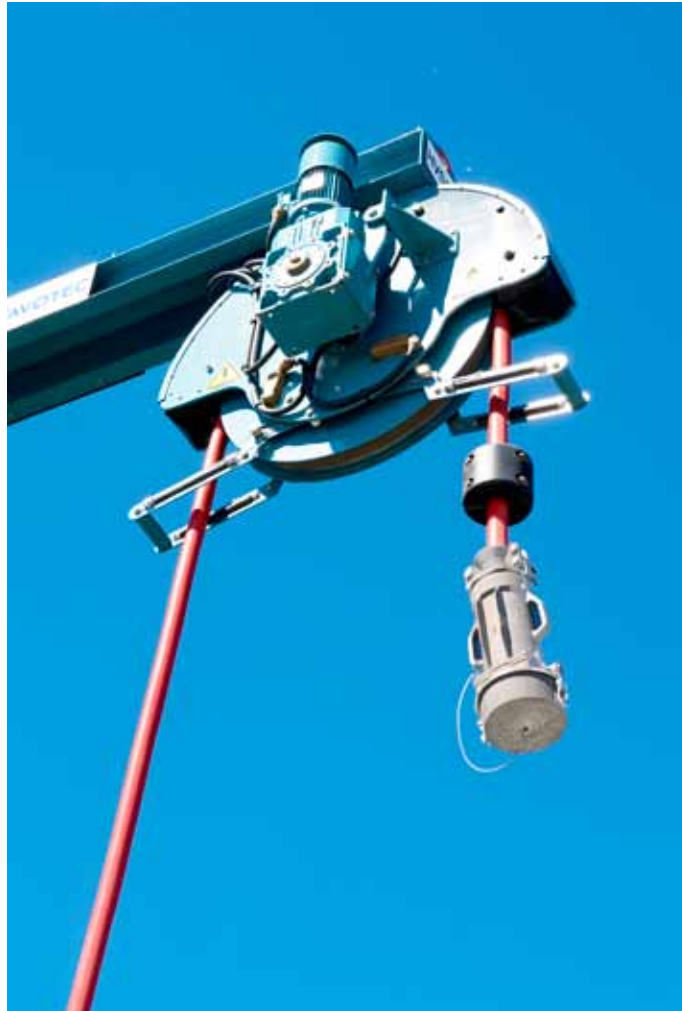
OPS-plug in the Port of Trelleborg.
