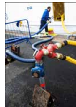
Components of Port Reception Facilities for ship sewage at the Port of Stockholm.
