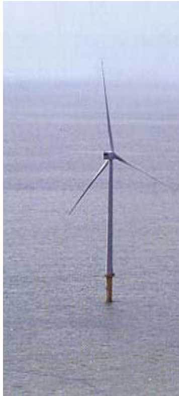
Figure 28 A Wind Generator
