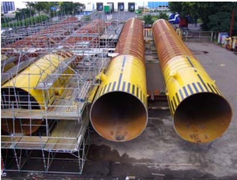
Figure 15 Typical underwater piping
