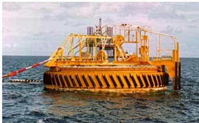
Figure 20 A Single Point Mooring buoy
