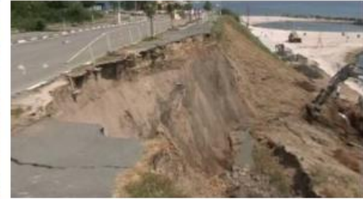
Fig. 3.5. c and d - Landslides under the promenade alley/sidewalk Eforie South
