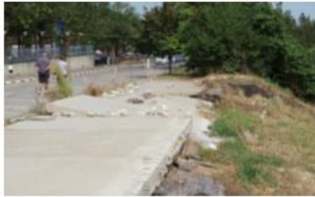
Fig. 3.5. c and d - Landslides under the promenade alley/sidewalk Eforie South
